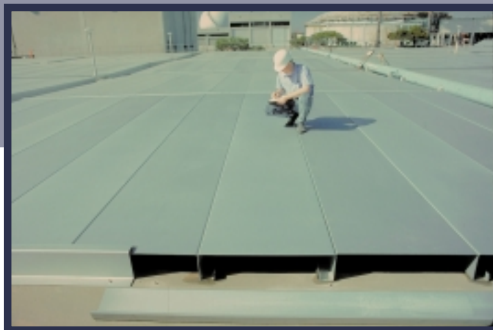
County Sanitation Districts, Orange County, USA ,Flat Covers for Sedimentation Basins.
