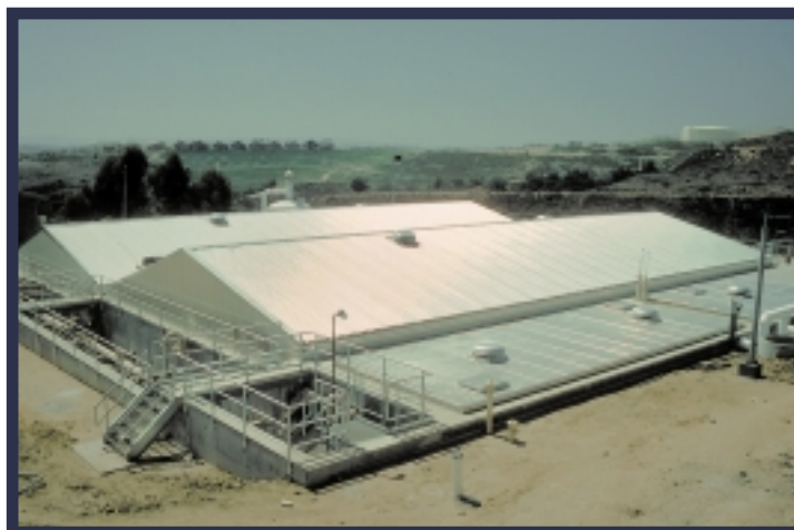
Trabuco waste water treatment plant, USA Batch reactor, truss roofs and aerobic digesters.
