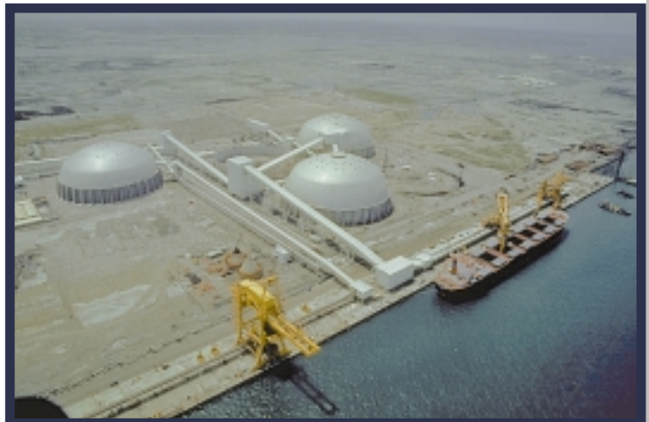
Completed 393' (120m) bulk storage domes after completion at FPC in Taiwan.
