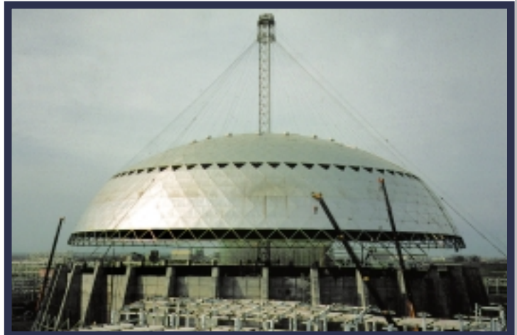
Bulk storage dome 393' (120m) under construction at FPC in Taiwan.
