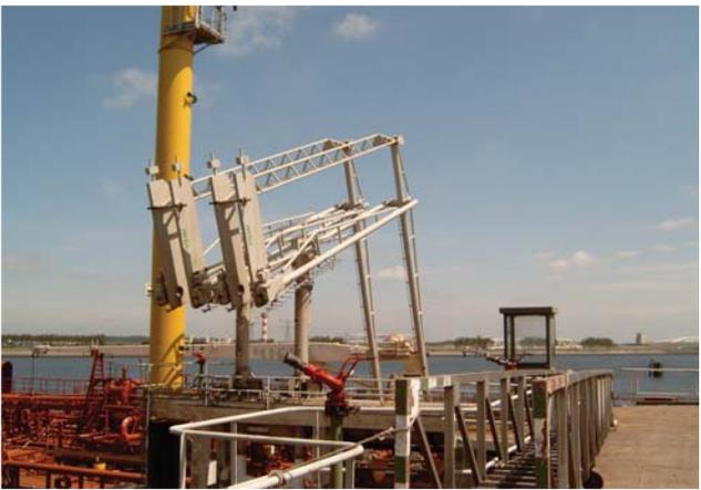
The MLA260 series is the most efficient range of marine loading arms on the market, due to the slim design and the availability of a number of design options to ensure that specific site requirements are met in the best possible way.
