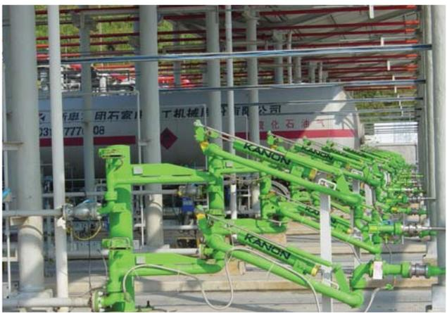
The advantage of Bottom Loading Arms is that these can be operated at ground level without need for loading platforms.
