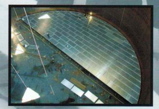
floating roofs, both for new installations as well as for retrofit applications. In recent years we have gained extensive experience converting external steel floating roof tanks to a tank design incorporating an aluminium dome roof covering an internal floating roof. Some of the projects we covered included cable suspended internal floating roofs, eliminating roof legs contacting the tank bottom.
