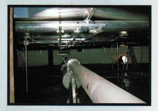
unwanted liquid. CTS supplies a complete range of floating suction units from 2" to 30", designed for horizontal and vertical tanks, accommodating fixed and floating roof tanks. Used materials include aluminium, carbon steel and stainless steel.
