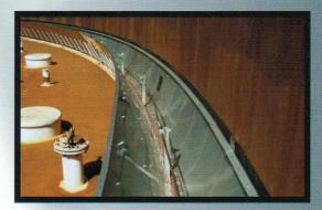
trapping water and product in the area directly behind the rim. Apart from reducing corrosion of the floating roof, an integral foam dam reduces the quantity of foam required for fighting a rim fire significantly, as the space to be filled with the foam is drastically reduced.
