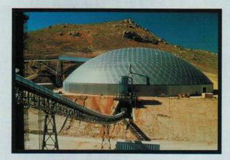
minimal costs, shielding the stored materials from the elements and protecting the direct neighbours from bulk materials getting dispersed by the wind or drought. Apart from these important dome features, the domes will require no future maintenance and will also reduce spraying efforts drastically.
