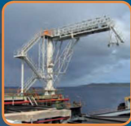
Column with telescopic gangway, stowed parallel to the berthing line. Valdez - Alaska
