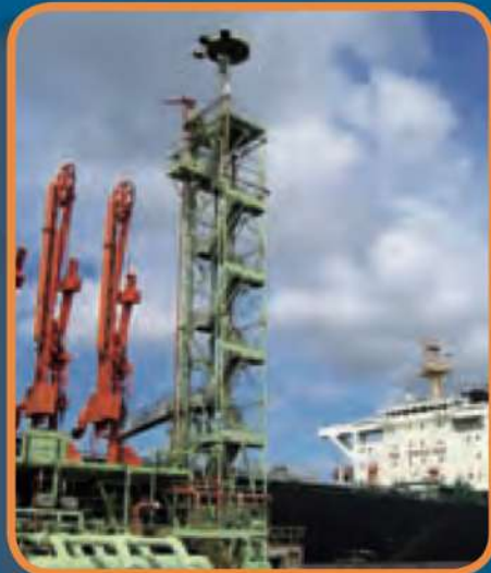
Gangway tower with floodlight support. Curacao - Dutch Antilles
