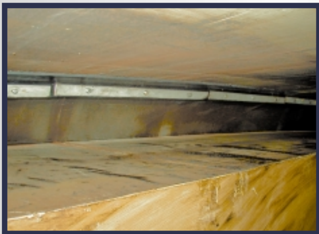
Bottom view of the primary part of a CTS40 double compression plate seal after installation, this particular seal was executed with a double flipping tip to bridge a nominal rim gap of 350mm (14")!
