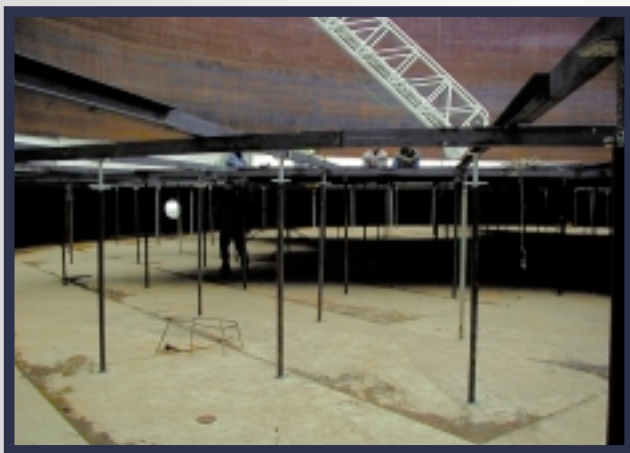
Cable suspended roof (no legs), top and bottom view.
